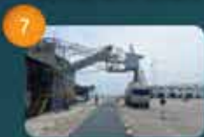
Terminal Semen Apung Kuala Tanjung, Sumatra Utara Kuala Tanjung Floating Cement Terminal, North Sumatra
