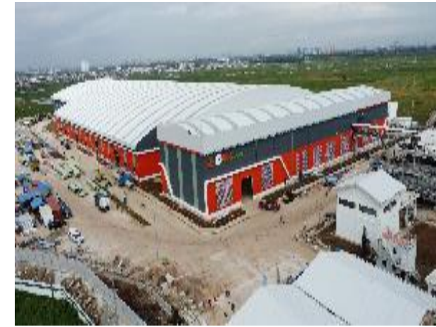
RDF Rorotan Facility
