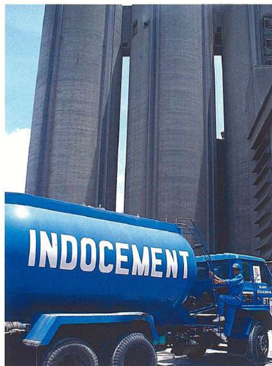
Left: Cement is stored in concrete silos at Indocement's production facilities.
