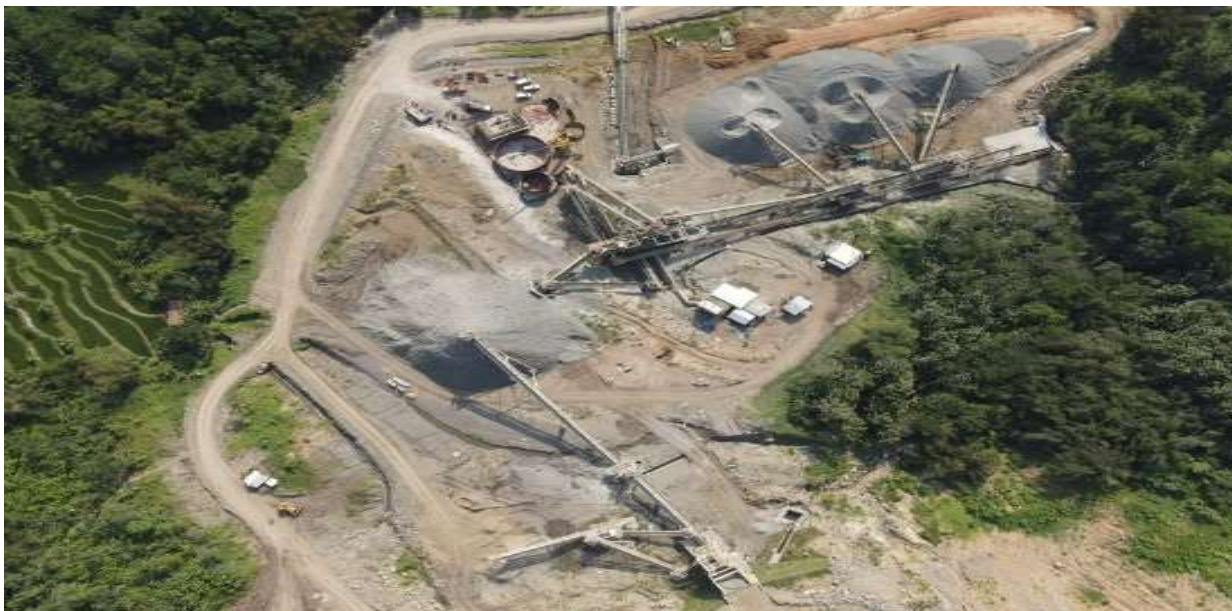
Crusher & Washing Plant Area
